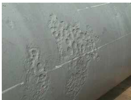
Fig. 1 – Defective type of loss of material caused by corrosion.
